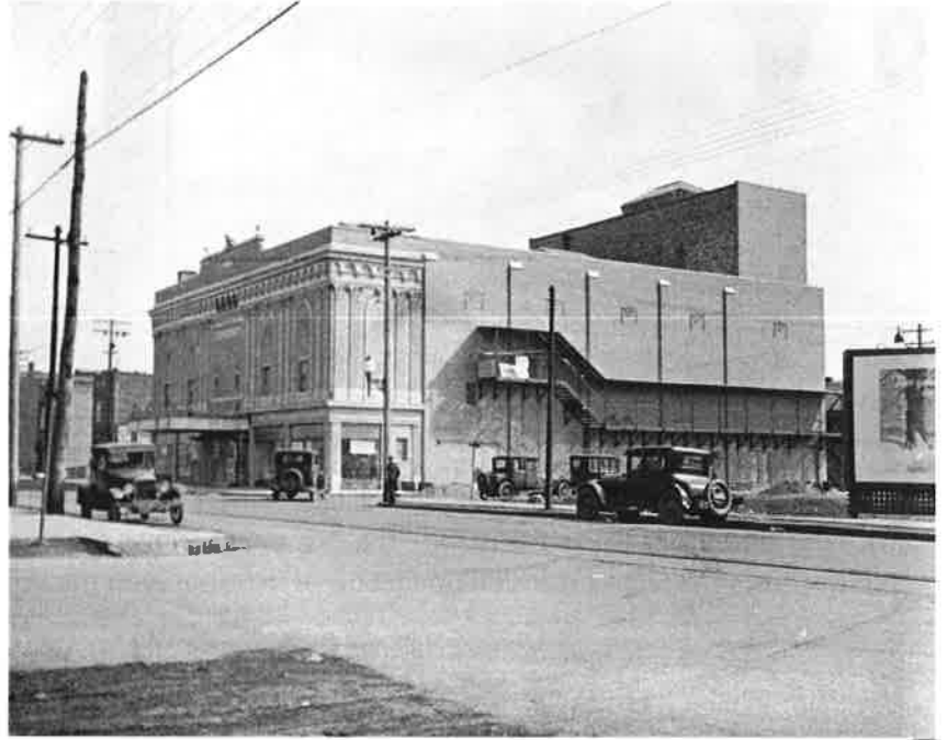
Looking east from north side of Jericho Turnpike - The Glynne Theatre (eventually the Floral Theatre) just after its construction.
